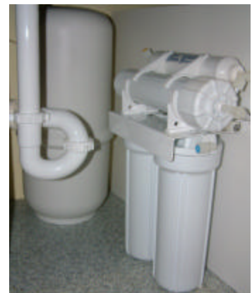
Installation under sink
