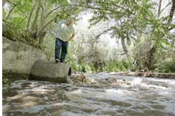
CHARLIE NEUMAN / Union-Tribune Superintendent of the Escondido Canal Carl Burgess watched with pleasure yesterday as water flowed again, here from the outfall pipe directing water to Lake Wohlford. Six of 13 miles was blocked by mud and rock during December and January's heavy storms.
